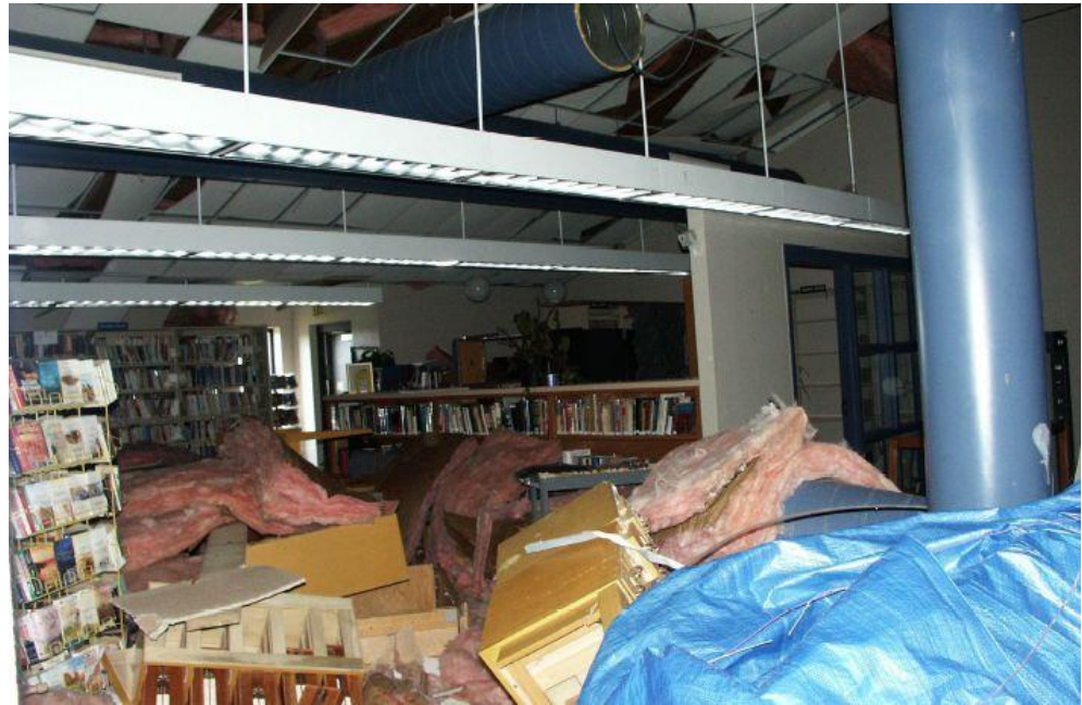
Interior of the library after the tornado hit
